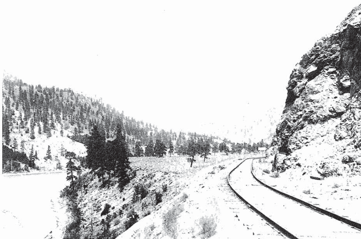
FIG. 15. A view up the Thompson River taken in 1885 at the completion of the CPR in B.C. Drynoch station can just be seen at the foot of the cliff. The profile of Drynoch landslide, approximately 2 km to the north, appears just above the station (B.C. Archives photo 74995).
