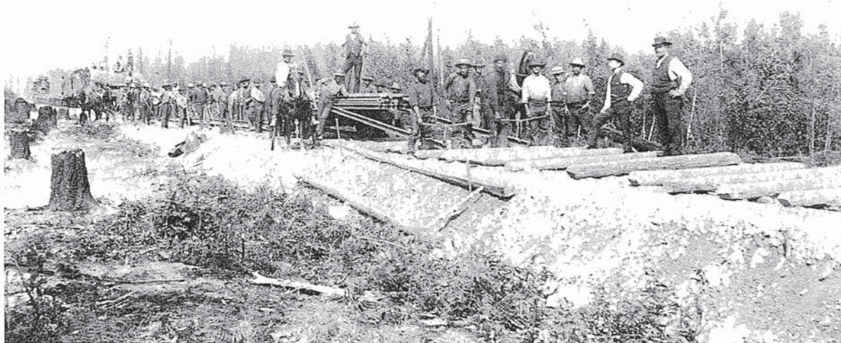
FIG. 14. An 1881 photograph of the construction of the CPR, presumably taken close to the construction camp shown in Fig. 13 (B.C. Archives photo 75116).
